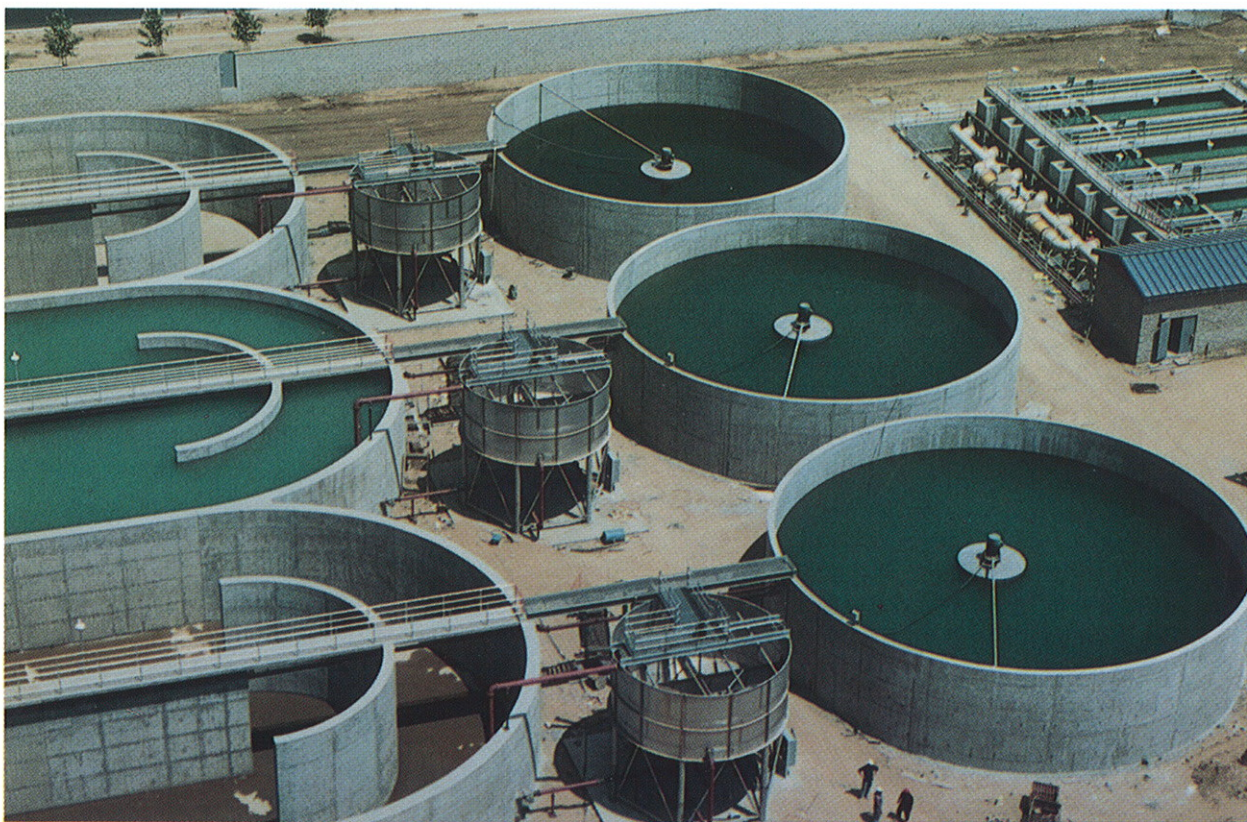
The wastewater and reclamation facilities for the Chino Basin Municipal Water District in California will incorporate the SAC™ bio-control system to maintain a constant sludge age. This plant will ultimately handle a flow rate of 28 mgd of both domestic and industrial wastes. The system also utilizes other innovative treatment processes such as the NITROX® ORP denitrification process, the BOAT® intra-channel clarifiers, and the BULLSEYE® nutrient removal process.
