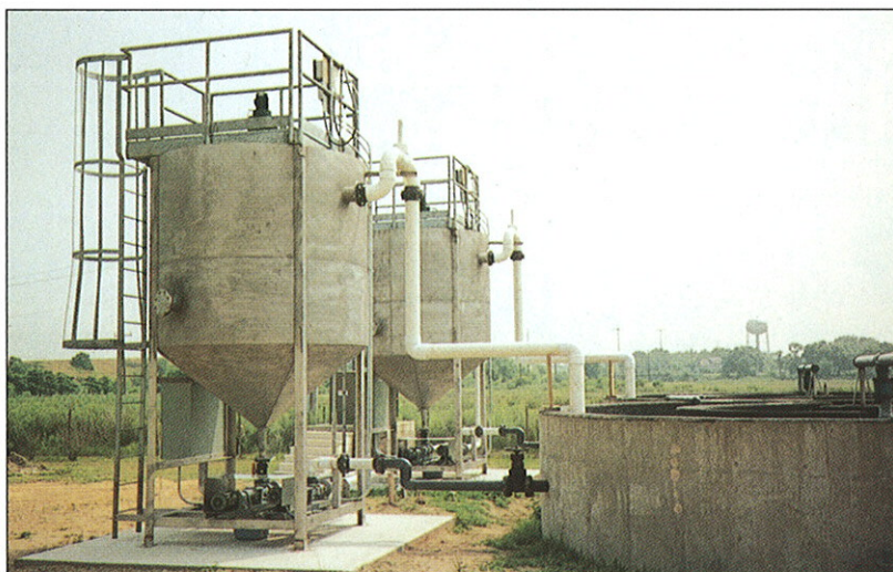
This 0.75-mgd wastewater treatment plant in Lewes, DE, operates two aeration basins with dual SAC™ Bio-Control Units.
