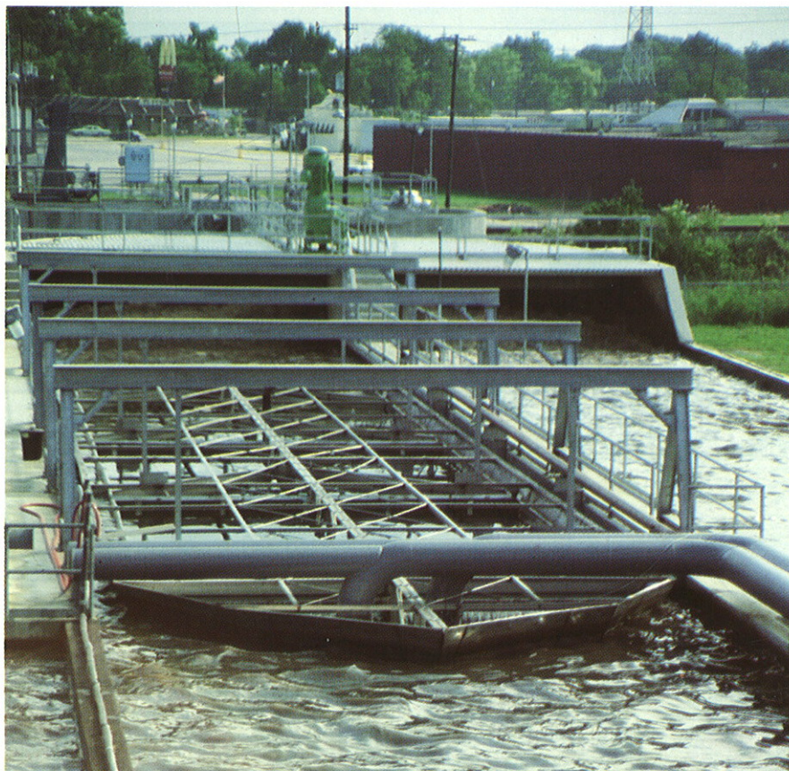
The BOAT® clarifier's suspension structure and the motor for the vertical turbine aerator are seen in this close-up.
