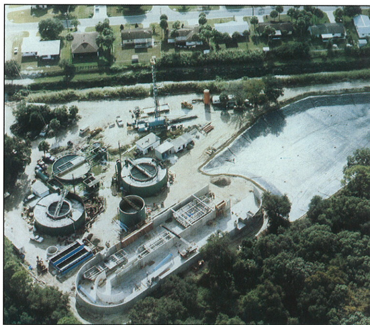
Figure I The end of the oxidation ditch can be left open to allow trucks and cranes to drive into the basin for easy installation. The existing treatment plant can be kept in operation while the new facilities are under construction. The oxidation ditch and BOAT ® clarification system can also be incorporated with a unique odor control system, which is especially important when homes are in close proximity to the plant site.
