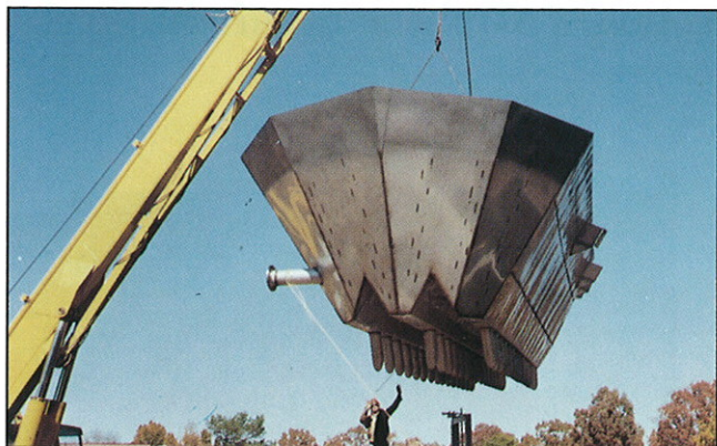
Figure E For smaller facilities, the clarifiers are shipped to the jobsite as a single unit. Thus, each unit can be easily lifted off the truck and suspended in the ditch.
