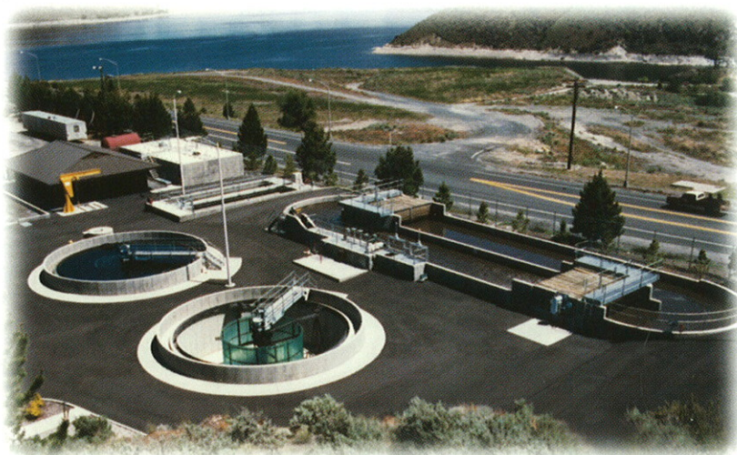
The oxidation ditch facility at Grand Coulee, Washington was retro-fitted with the NITROX™ denitrification system. Lower SVI values and reduced energy costs were achieved, along with reductions in the Total Inorganic Nitrogen (TIN) effluent levels.
