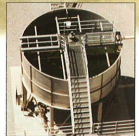
Automatic Sludge-Age-Control was accomplished at a large water reclamation facility in California which will ultimately treat 28 mgd. Sludge at this facility is dewatered using centrifuges and is then transferred to a composting facility.
