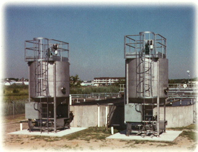
This facility in Delaware was retro-fitted with twin bio-control units – one for each aeration tank. Plant down-time was minimal and the manpower requirement for sludge handling was reduced.
