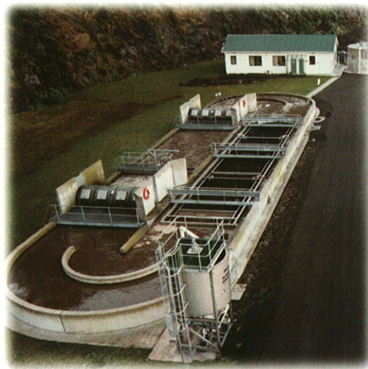
Twin oxidation ditches were utilized to add capacity and upgrade an existing activated sludge/RBC facility. This 1.5 mgd (5678 m 3 /d) system utilizes a single SAC™ bio-control unit for each ditch. Thickened sludge is continuously pumped to aerated holding/digestion tanks. This system allows for the sludge to meet Class B requirements.
