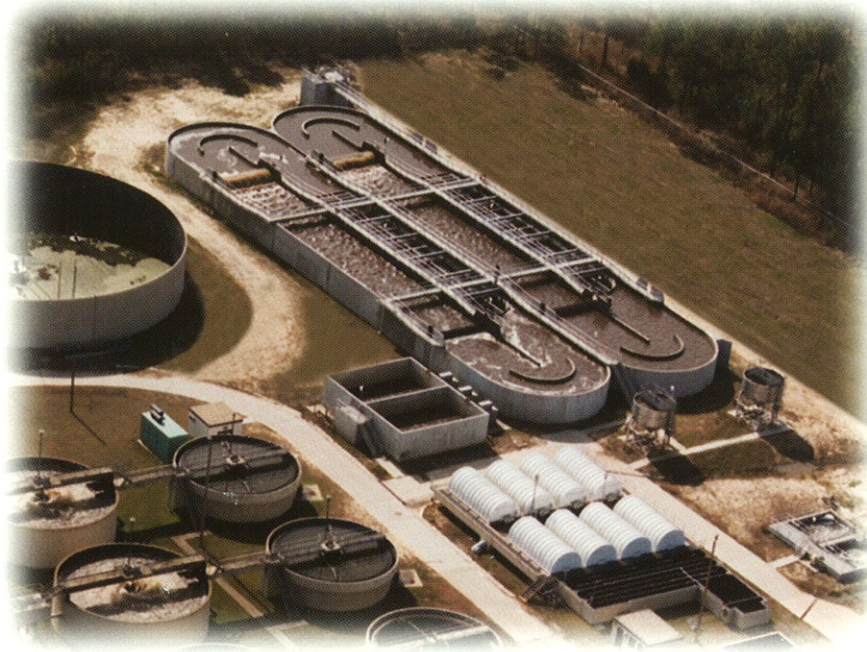
Twin oxidation ditches were utilized to add capacity and upgrade an existing activated sludge/RBC facility. This 1.5 mgd (5678 m 3 /d) system utilizes a single SAC™ bio-control unit for each ditch. Thickened sludge is continuously pumped to aerated holding/digestion tanks. This system allows for the sludge to meet Class B requirements.
