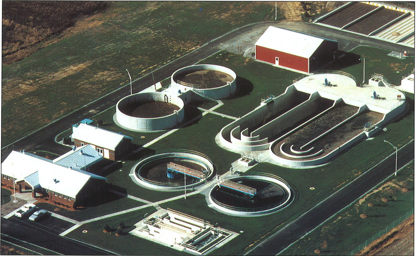
Aerial view of the treatment plant in Sellersburg, Indiana featuring oxidation ditches with SIMCAR® vertical turbine aerators.
